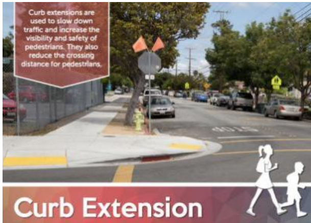
Curb Extension: Example of Traffic Calming Measure viii
